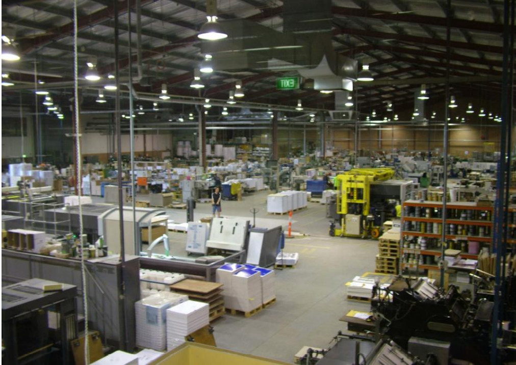
LED lighting in production area
